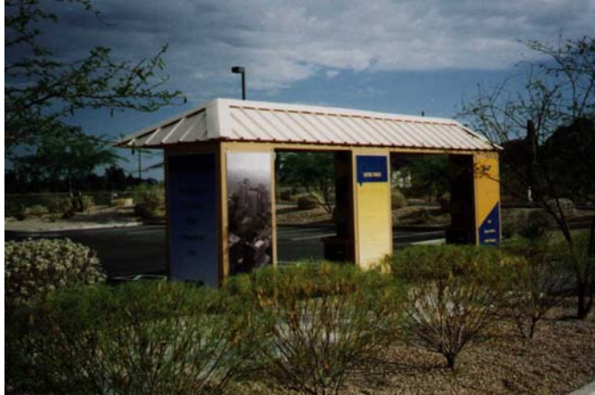
Figure 5-18. Public charging station with informational graphic panels.
